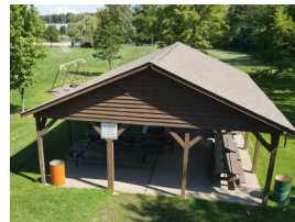
Near Railroad Tracks
